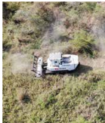
Mechanical ground preparation in Nyinkuac
